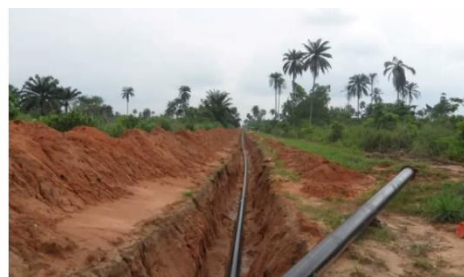
Temporary construction slope
